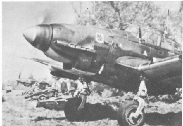
Below: Ju 87D in Russia, summer 1943. Note that the aircraft is painted in conventional splinter camouflage all over—unusual for this type of unit—and that the badge of 7 Staffel, Stukageschwader 1 is marked on the cowlings. The rims of the machine gun ports in the wing leading edges are painted yellow.
